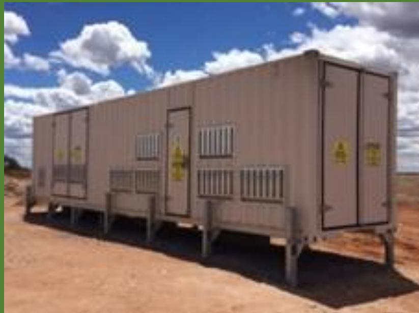
Preassembled inverter stations were placed on rammed supports. One inverter station was placed per “power block” (39 in total).
