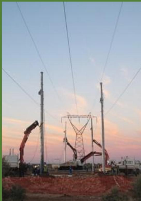
In order to feed electricity into the existing 132kV ESKOM power line from the 75MW solar facility, a tie-in was necessary from the newly built sub-station. A multitude of civil and structural work had to be completed in time to successfully connect to the ESKOM grid within a limited time due to the pre-arranged shut-down
